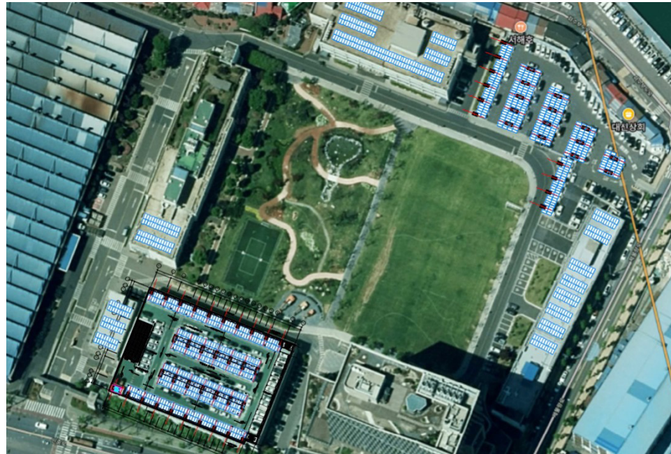
* Planned location of the Incheon plant's solar power plant
